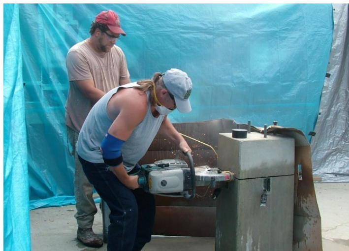
Sparks fly as Sam cuts through some rebar during the pier cut. Ted sprays down the blade to minimize dust and blocks concrete slurry with a piece of cardboard. Sam & Ted work for Stover Construction who donated the pier cut for our new 16" telescope installation.
